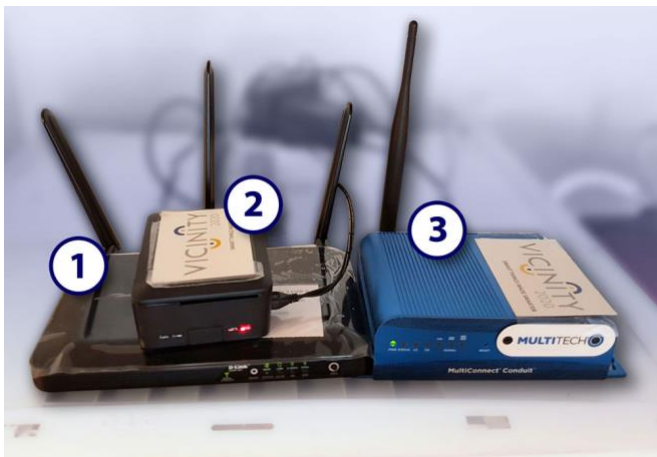
Figure 8: Routers/gateways placed on top of the refrigerator
